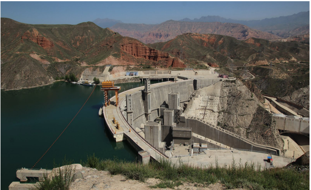
Lijiaxia Hydropower Dam in Kamra National Park, Chentsa (Ch: Jiancha) County, Qinghai Province. 2013 ©RD
