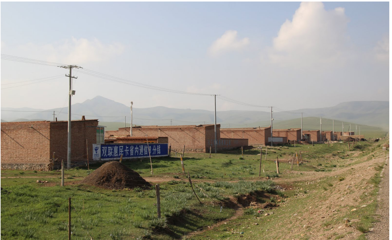
Resettlement housing near Sangchu (Ch: Xiahe), Kanlho (Ch: Gannan) Tibetan Autonomous Prefecture, Gansu Province. 2013 ©RD
