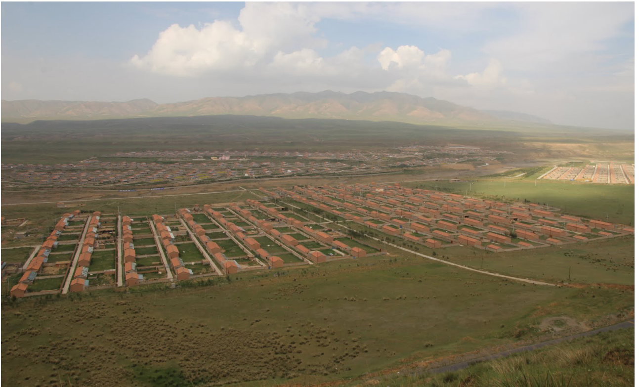
Resettlement housing near Baima, Golok (Ch: Guoluo) Tibetan Autonomous Prefecture, Qinghai Province. 2013 © RD
