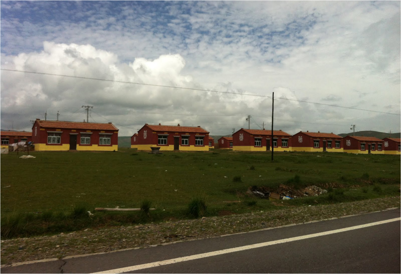
Resettlement housing near Gepasumdo, Tsolho (Ch: Hainan) Tibetan Autonomous Prefecture, Qinghai Province. 2013 © RD
